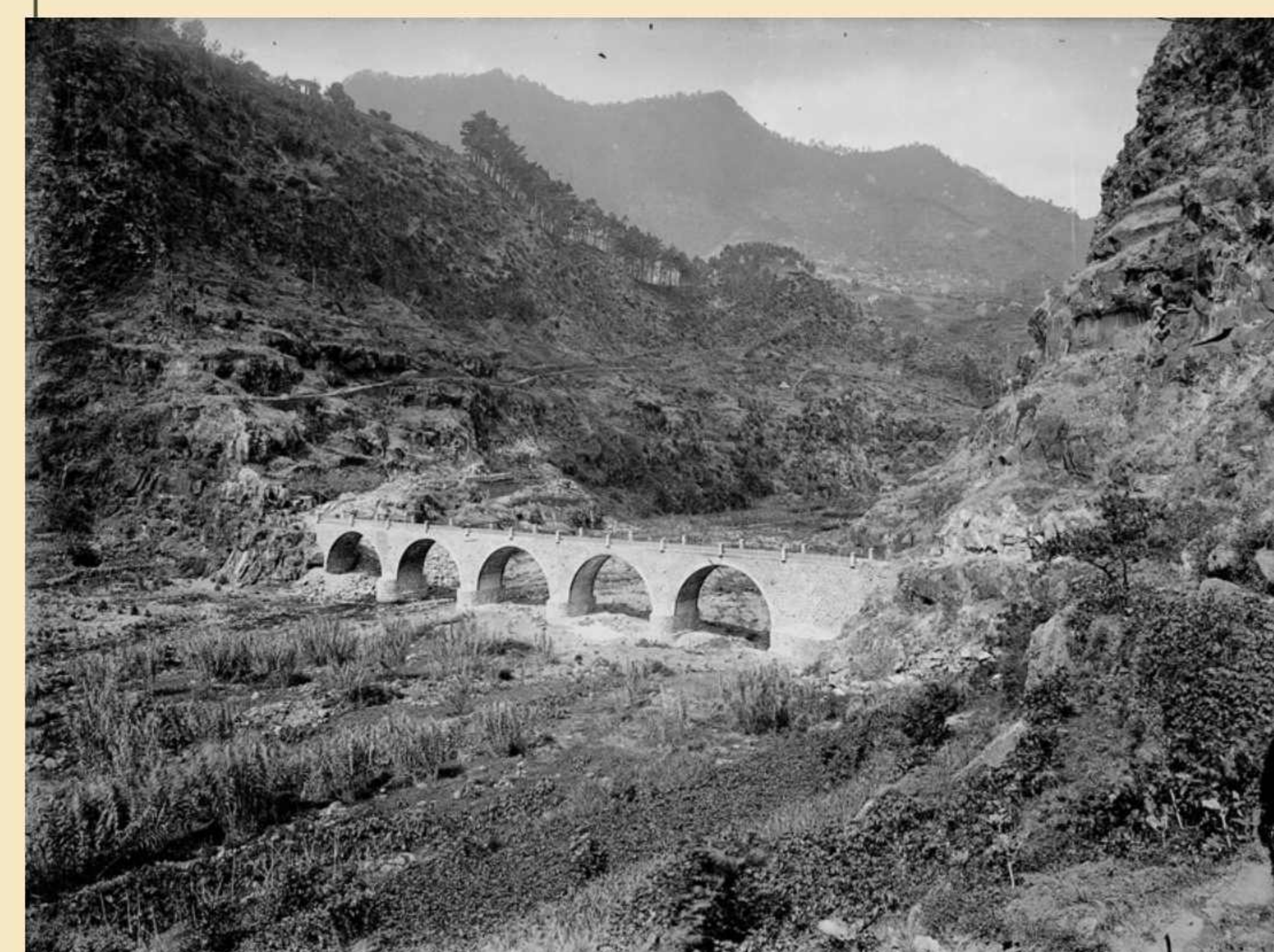
View of the bridge over the stream of Metade, from Molinhos area; one can see: the five arches and balconies on the deck of the stone masonry bridge and the construction works for the opening of the National Road 1 (currently Expressway 1); on the left, Lombo (high land) de Baixo and Pico (peak) areas; halfway up the hill, a section of the Royal Road 23. Photo by Perestrellos, 1910, glass plate negative, MFM-AV, in deposit at ABM, PER/242.
