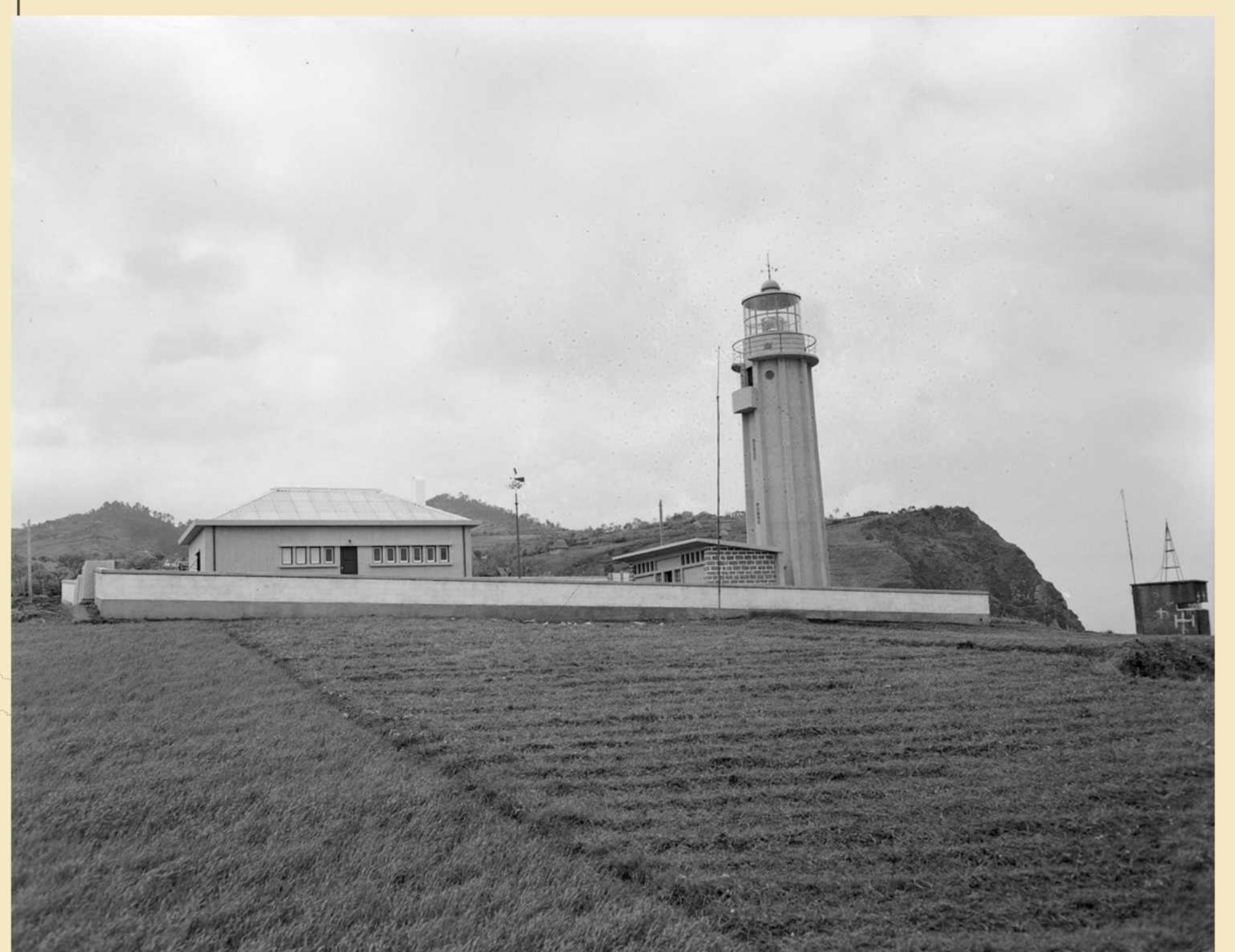
São Jorge lighthouse in Farrobo area; one can see: a wall bordering the lighthouse keepers' house, the compass rose in the courtyard, the electrical substation and the lighthouse crowned by a dome and a compass rose; on the right, an observation post and radio antennas. Photo by Perestrellos, 1959-03-31, film negative, MFM-AV, in deposit at ABM, PER/6906.
