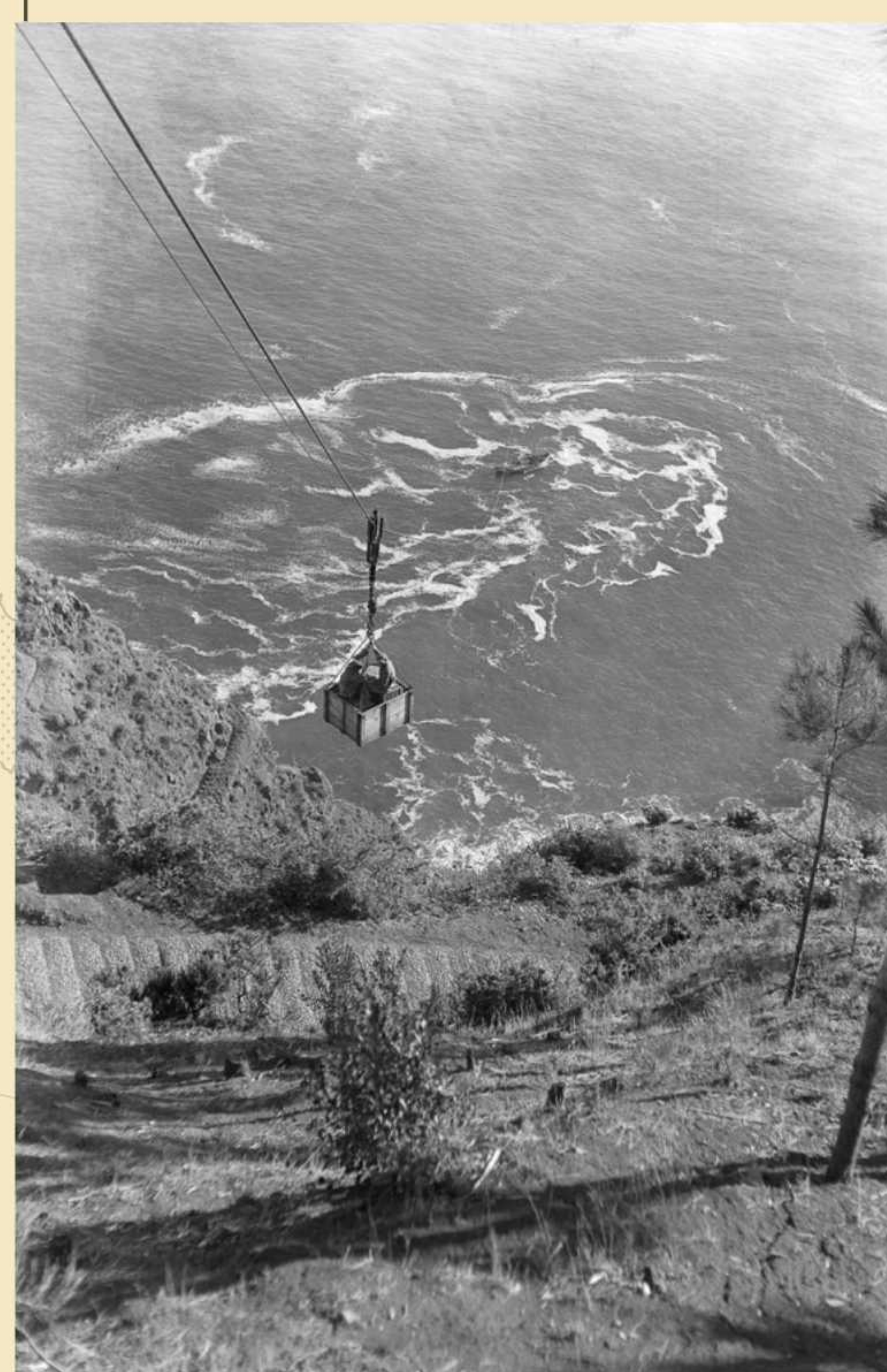
Aerial cableway (currently Cabo Aéreo viewpoint); one can see: a steel cable with one end attached to the seabed; a man and a boy in the wooden cargo box; in the sea, a cargo vessel at anchor; on the hillside, the cobbled steps of the Royal Road 23. Photo by Perestrellos, 1948-02-05, film negative, MFM-AV, in deposit at ABM, PER/6870.
