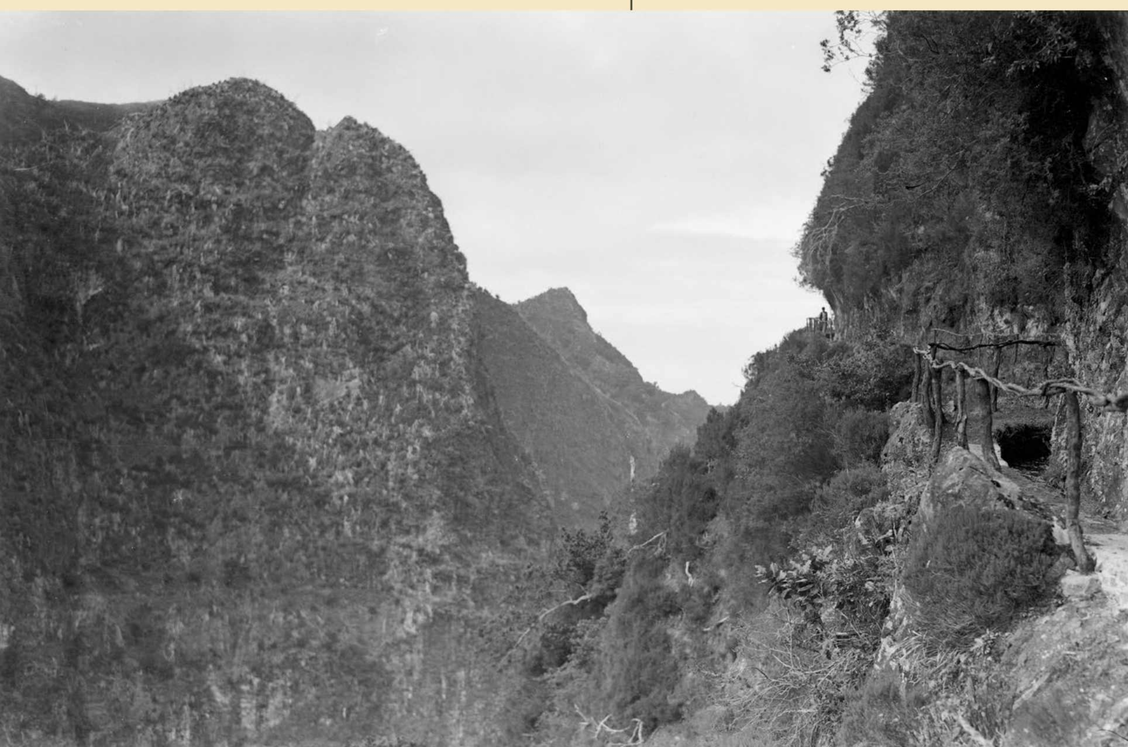
Caldeirão Verde "levada" (water channel). In Queimadas area; one can see, on the right, a wooden balcony, the "levada" carved into the rock and a man. Photo by Figueiras, post 1930, film negative, MFM-AV, in deposit at ABM, PHF/689.
