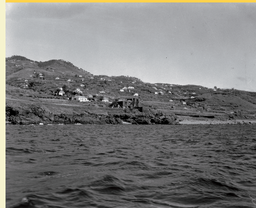
Seaview of Reis Magos, Caniço; revealing an old 18 th century building in an advanced state of ruin. Photo by Perestrelas, 1960s, glass plate negative, MFM-AV, in deposit at ABM, PER/7995.
